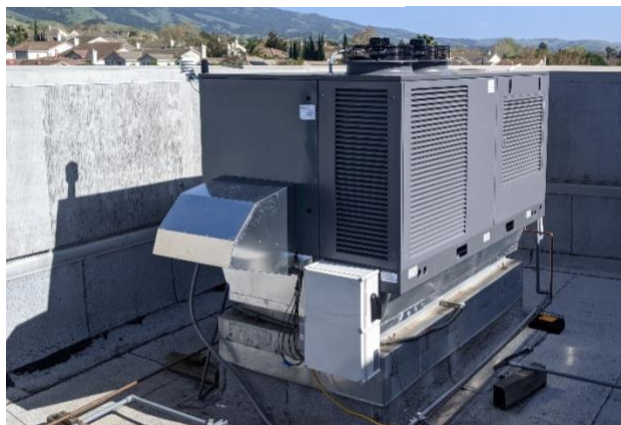
Figure 5. packaged heat pump with IDEC RTU
