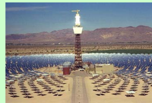
Solar Power Tower
